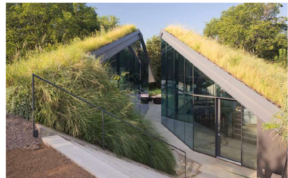
Figure 5: A green roof
